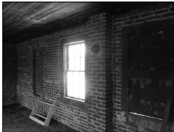
Interior of upper floor, visible: flue for one of four coal burning stoves
