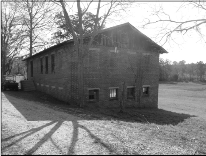
Hatchery building; Northwest view
